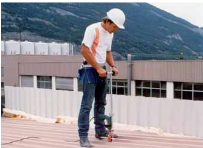
Fixing trapezoidal sheet metal using self-tapping screws
