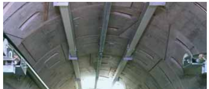
Curved HALFEN Cast-in channels in tunnel segments
