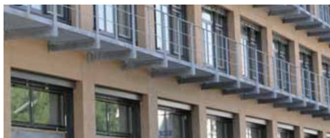
Fixings for emergency access balconies (Vertical installation of HALFEN Channels)
