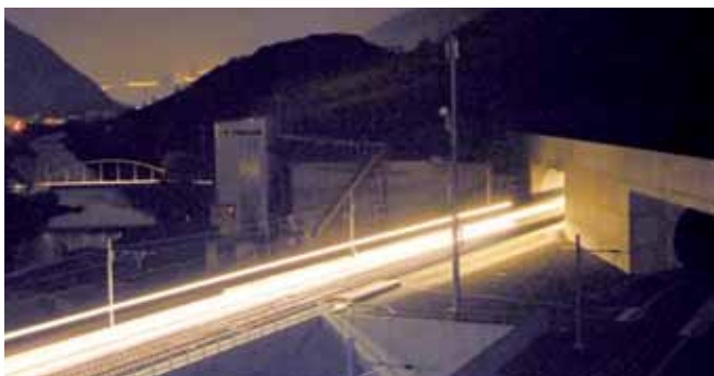
Lötschberg-Base tunnel, Switzerland
