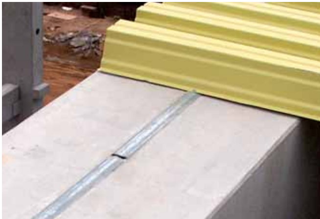
Fixing of trapezoidal sheet metal roofing
