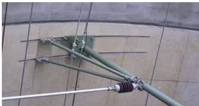
Fixing of overhead cables in railway tunnels
