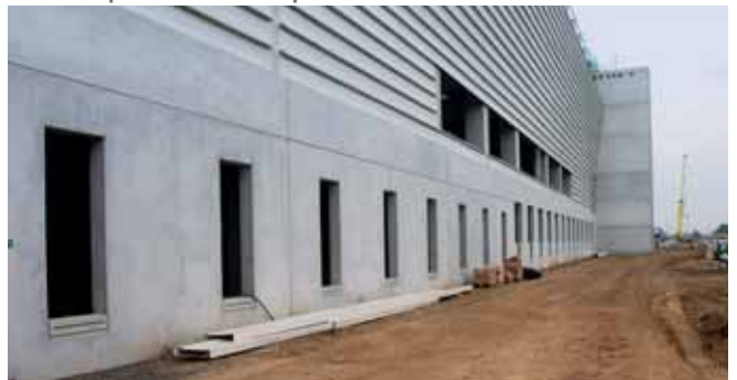
UPS Air Hub, Cologne Bonn Airport, Germany
