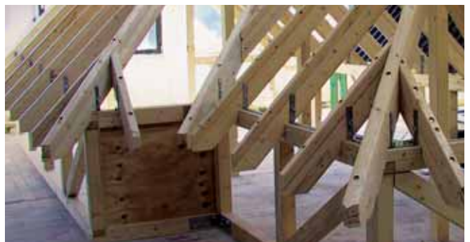
Timber pitched-roof construction
