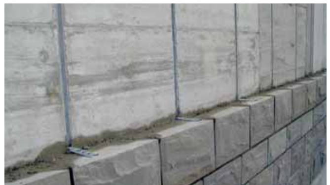
HALFEN ML Brick-tie anchor system
