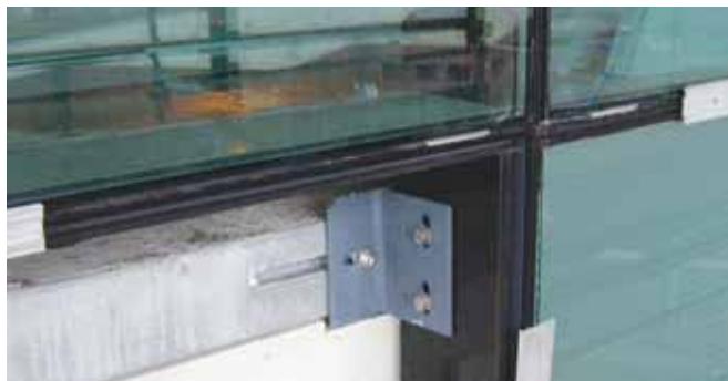
Fixings for curtain wall façades
