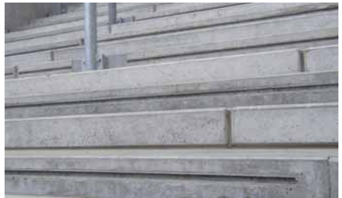
Fixing of safety rails, Rheinenergiestadion Cologne
