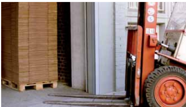
Corner guards in an industrial environment
