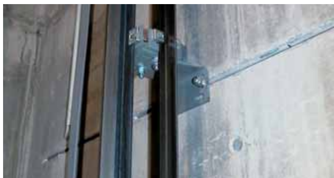
Fixing guide-rails with HALFEN Channels
