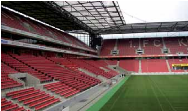
Fixing of safety rails, Rheinenergiestadion Cologne
