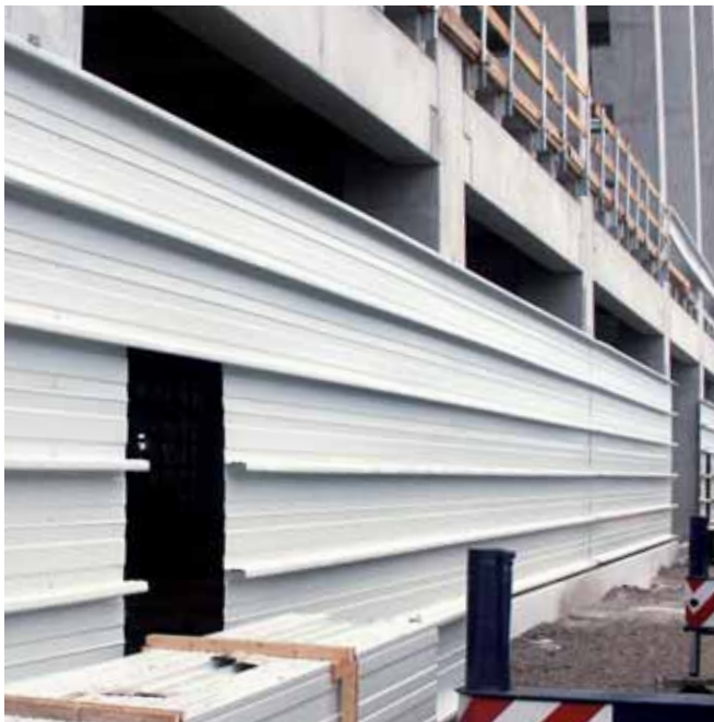
Façade fixed using HALFEN HTU Cast-in channels
