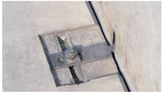
HALFEN HKZ Restraint tie with serrated washer
