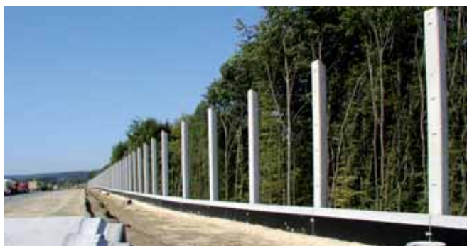
Fixings of noise barriers to concrete posts
