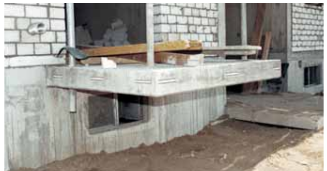
Cast-in HGB Channel, residential building
